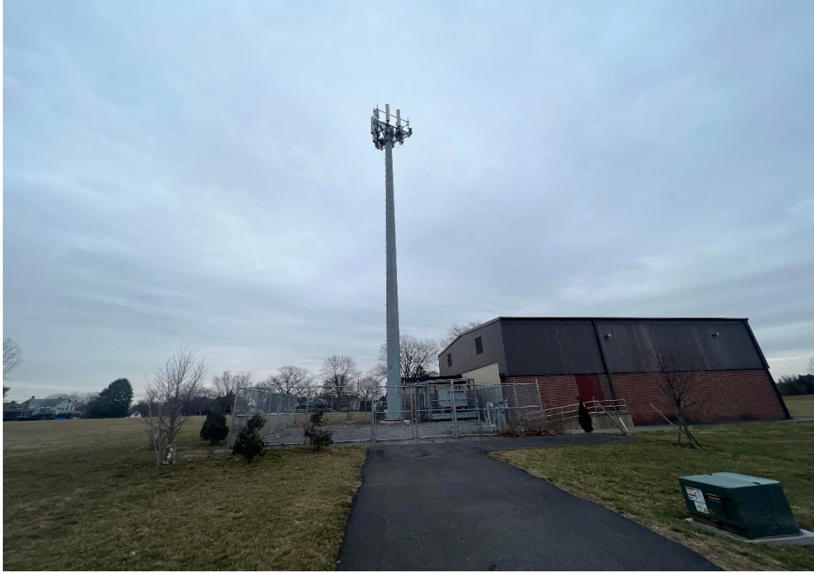
Monopole with Cell Antenna Installation
